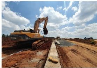
Phase II construction ongoing
