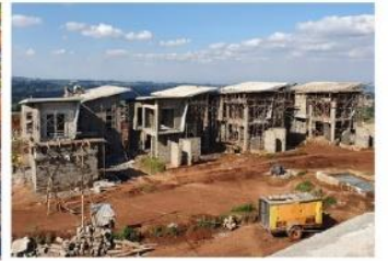
Ongoing construction of Tilisi Views
