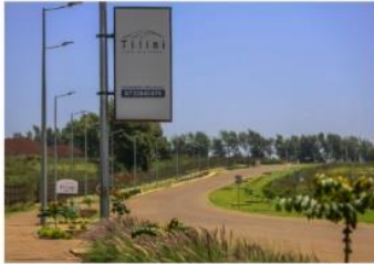
Completed Phase I infrastructure
